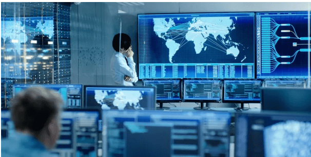
Command and Control Rooms
