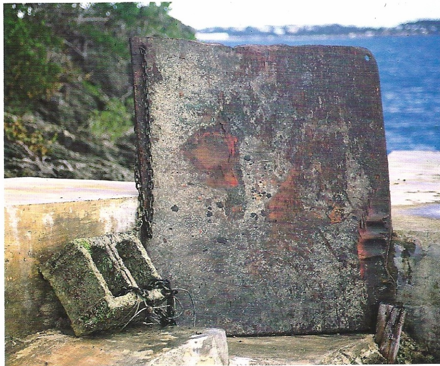
Urbanos, 1993 waterworks Urbanos, 1995 underside
