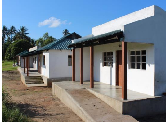
Finished houses ready for community outreach on resilient techniques.
