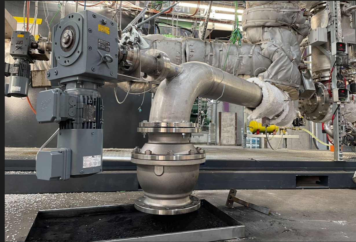
Fully automatic and continuous discharge for higher uptime and better ash quality.
