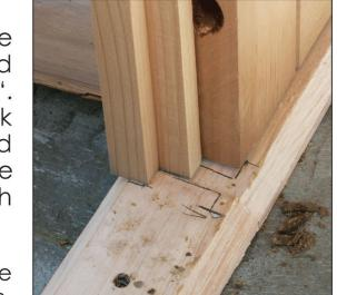
**Note:** When installing the wall panels and securing them to the posts using the 4" screws through the hole beneath the cross rail, remember to back the screw OUT one counterclockwise turn to allow parts room for expansion and contraction.
