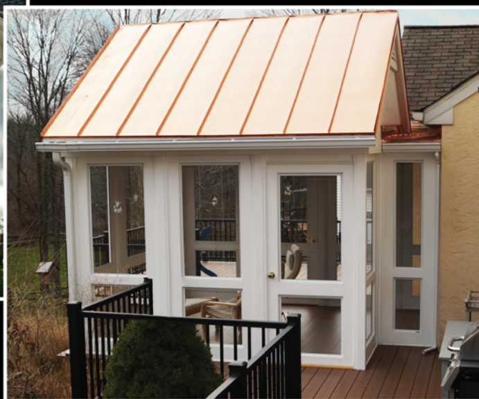
Above: porch with walkway attached to house
