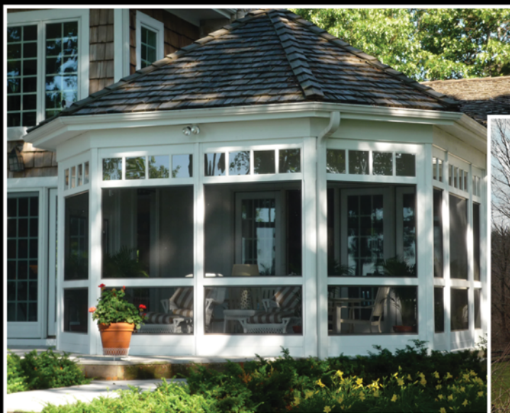
Above: New Construction porch with built-in transom glass
