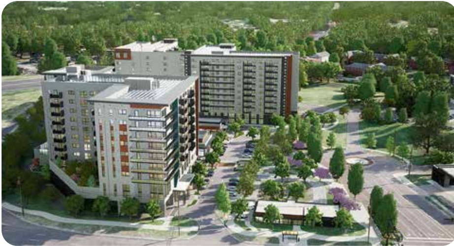
Lumina and Radia at Hillandale Gateway, nearing completion, will be the county's first zero-net-energy mixed-income project, providing 463 units, 54% affordable (30–80% AMI), alongside a regional transit center.
