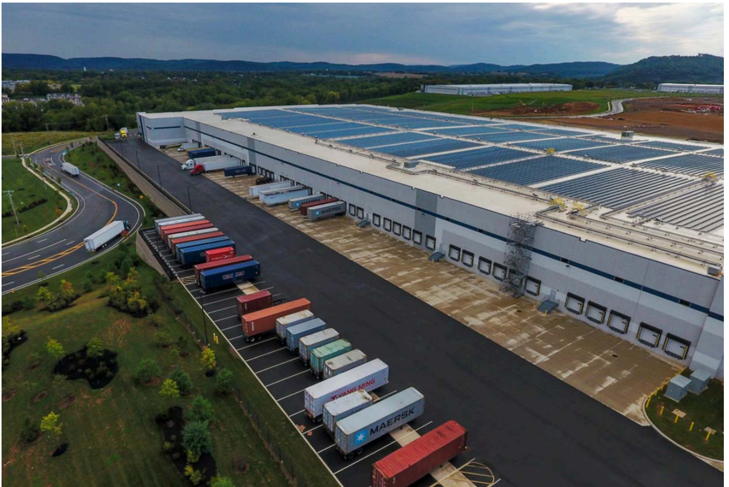
Solar panels unveiled Sept. 27, 2022, cover 1 million square feet of the Uniqlo distribution center in Phillipsburg, part of the Bridge Point 78 warehouse complex along Route 22 on the border with Lopatcong Township. Saed Hindash File Photo | For lehighvalleylive.com
