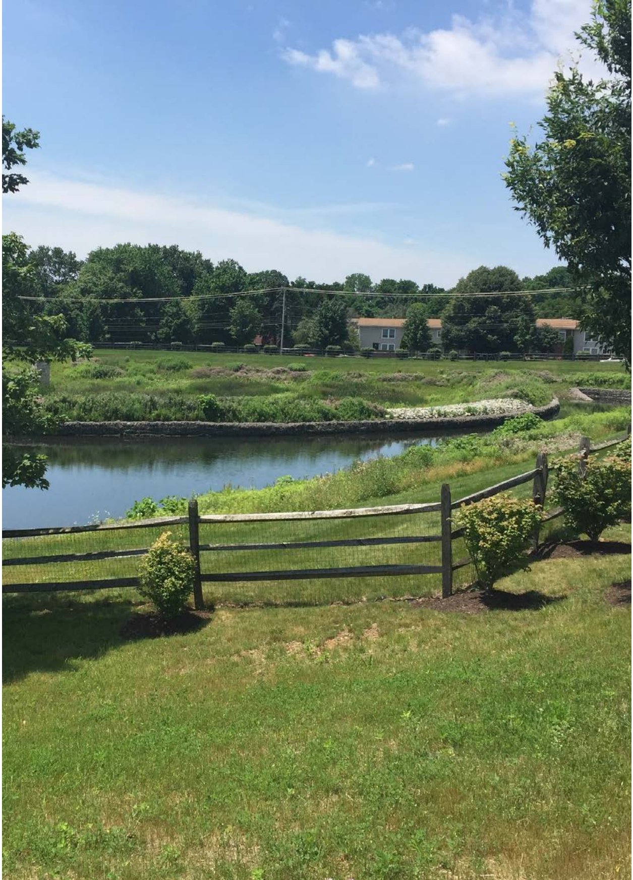
Wet pond/retention basin , photo by Craig Kackenmeister, LVPC
