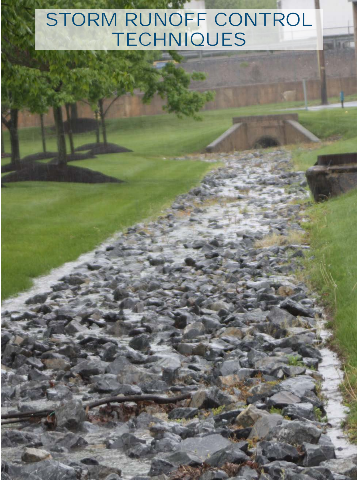
Rock-lined swale near intersection of Brodhead Road and Christian Spring Road, photo by Craig Kackenmeister, LVPC
