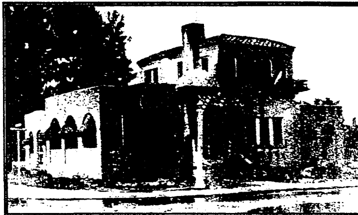
Figure 9 Shown as originally constructed at the northeastern corner of Washington Avenue and Espanola Way (currently the site of the Cameo Theatre), this circa 1926 Mediterranean Revival building was moved to its present site at 1745 Jefferson in June of 1938. The round arches were replaced with flat arches, and new porches were added sometime after its relocation (see recent photo in Figure 11).
