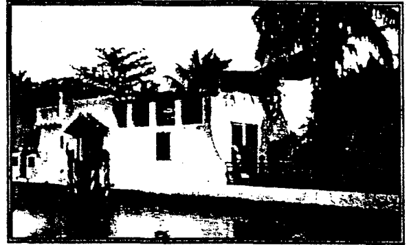
Figure 8 Constructed in 1925 and designed by Schultze and Weaver, this canalfront building located at 1818 Michigan Avenue was occupied by Henry Salem Hubbell from 1930 until 1940.
