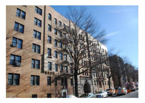
**EXTERIOR RESTORATIVE WORK**, including complete parapet reconstruction, selective profiled cast stone repair and reconstruction, selective windowsill and window lintel replacement as well as face brick repairs and replacement.
