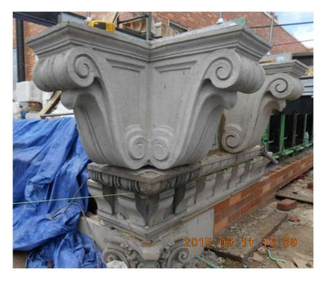
**HISTORICAL EXTERIOR RESTORATIVE WORK**, including dismantling decorative and salvaging terracotta cornice units for reinstallation and/or replacement with glass fiber reinforced concrete units to match the original terra cotta.
