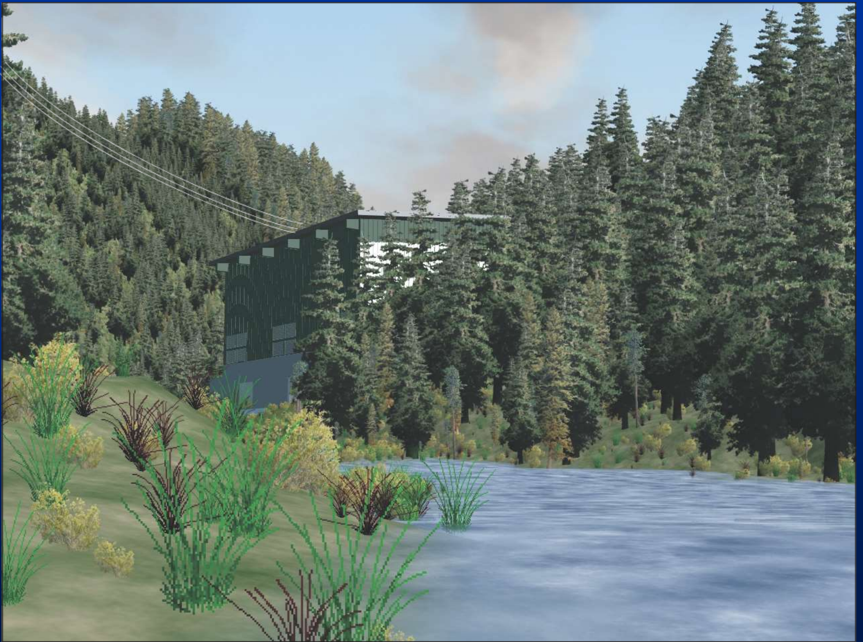
Powerhouse – 3-D model imported into VNS by RDI for Run-of-River Power Project 34
