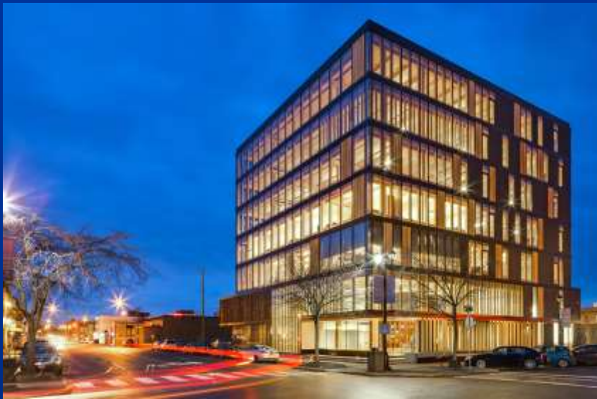
Wood Innovation and Design Centre – Prince George BC. Primarily Cross Laminated Timber. Credits: Ema Peter
