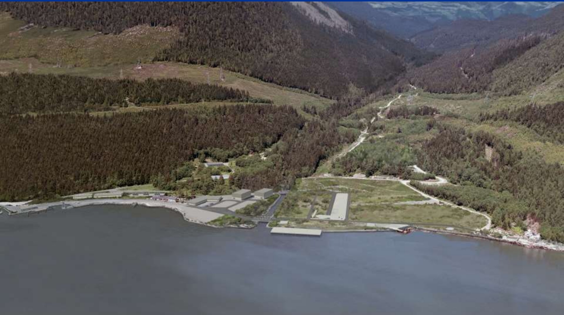
Simulation of Proposed Woodfibre LNG Facility single full 3-D Model in Photo to compare with VNS next slide – alternate viewpoint assessment difficult and expensive Source: AMEC 2016
