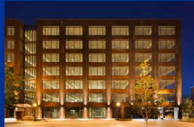
T3 Building Minneapolis – 3600 m 3 (1526 m 3 ) beetle killed Nailed Laminated Timber – 3600 T CO 2 captured over lifetime – largest in USA. Credits: Ema Peter
