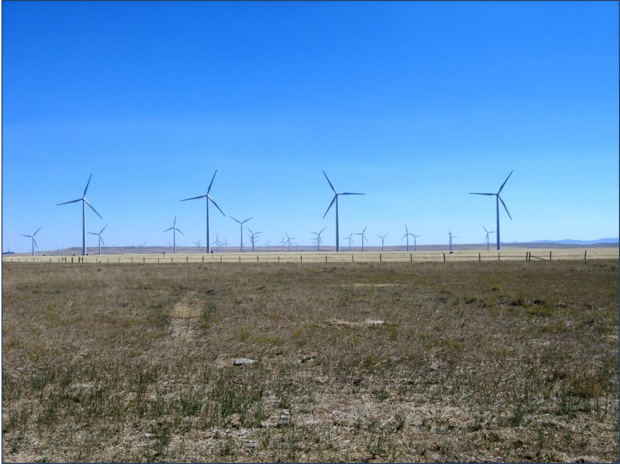
Figure 9 1.5 MW wind turbines, part of a 220-turbine wind farm near the town of Peetz in northeastern Colorado. In the western U.S. wind projects may include up to 1,000 turbines.
