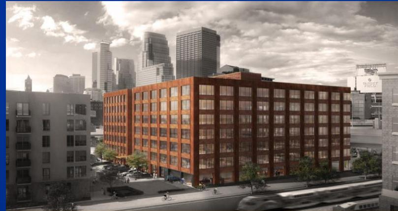
T3 Building Minneapolis – 3600 m<sup>3</sup> (1526 m<sup>3</sup>) beetle killed timber – 3600 T CO<sub>2</sub> captured over lifetime – largest in USA
