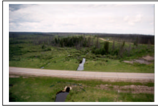
Highway buffer near Jacos plant
