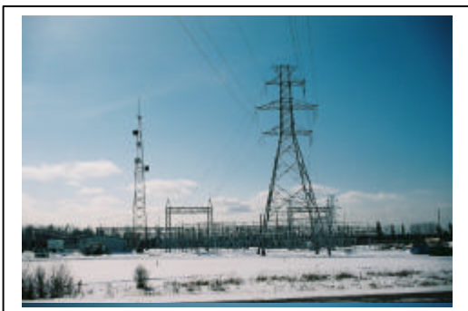
Hydro lines along Highway 63
