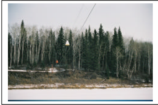
15-24 Cable crossing on Clearwater River
