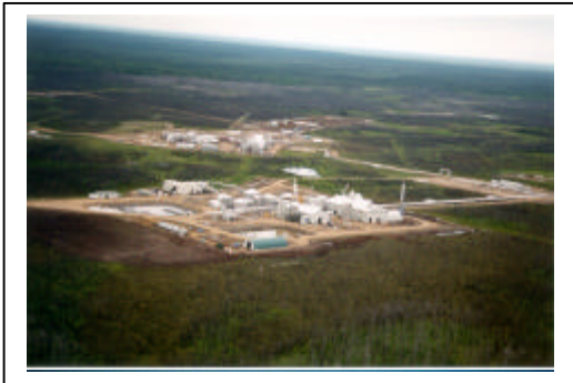
Jacos plant near Highway 63 (aerial view)
