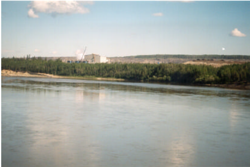
Structure near the Athabasca River
