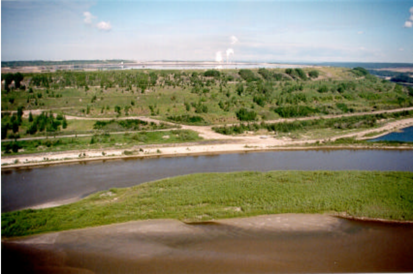
Re-vegetated containment structure
