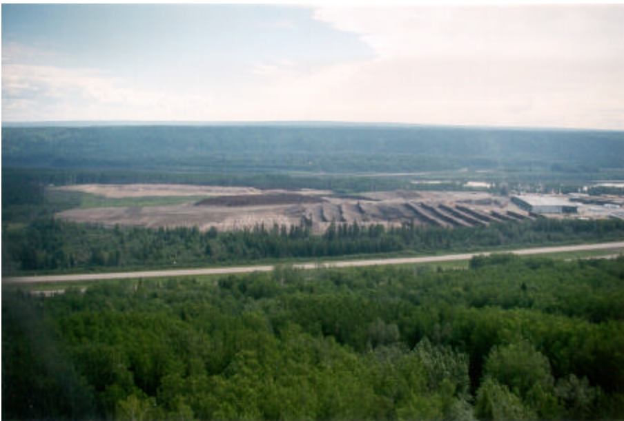
Northland Mill adjacent to Highway 63 and Athabasca River
