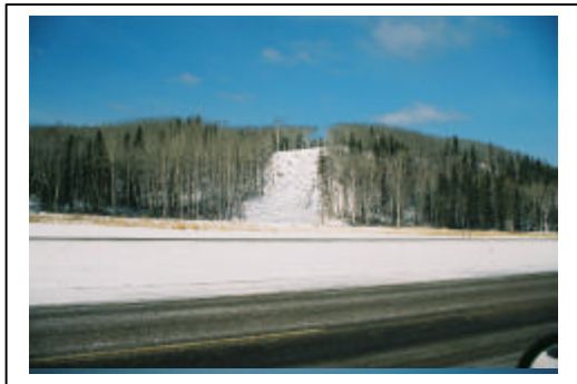
8-8 Pipeline along Highway 63
