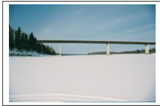
16-5 Highway Bridge on Athabasca River
