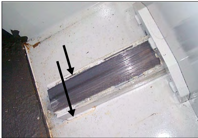
Figure 3-44 Tack weld on both sides of the floor guide
