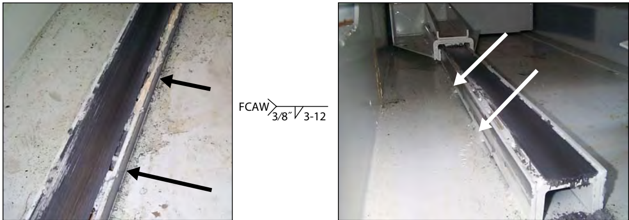
Figure 3-46 Welds on both sides of floor guide
