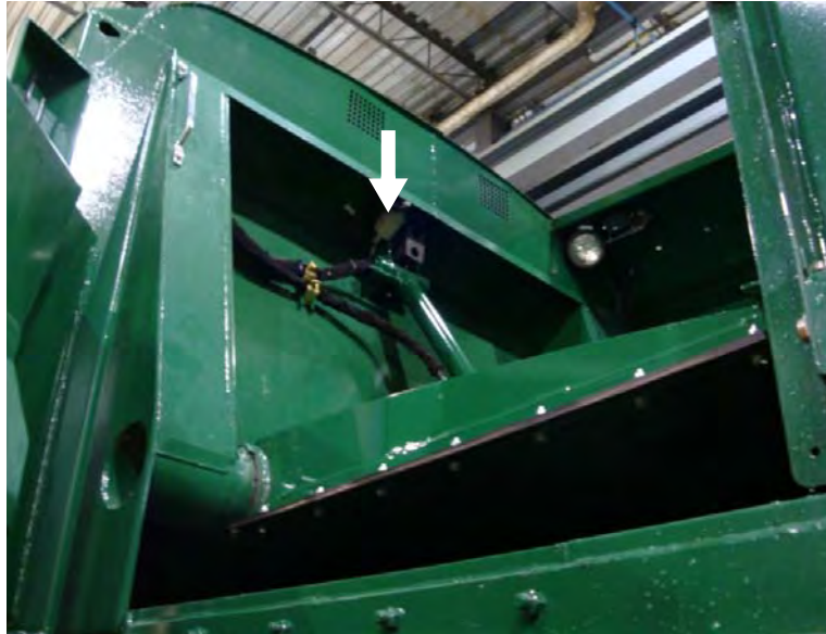
Figure 3-91 Crusher panel up limit switch
