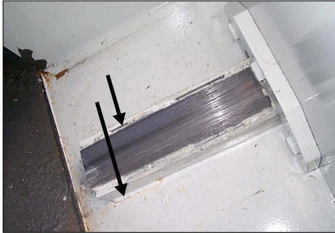
Figure 2-28 Welds on both sides of the floor guide
