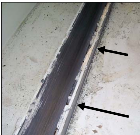
Figure 2-31 Welds on both sides of the floor guide
