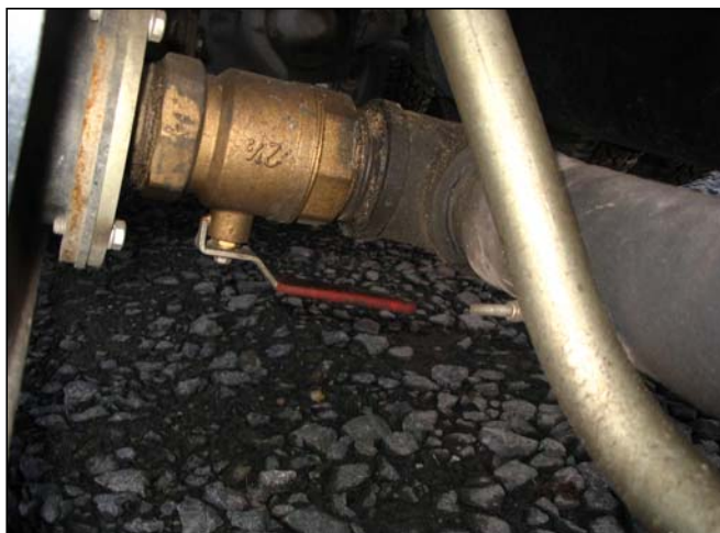
Figure 2-11 Suction line mounted valve (steel tank)
