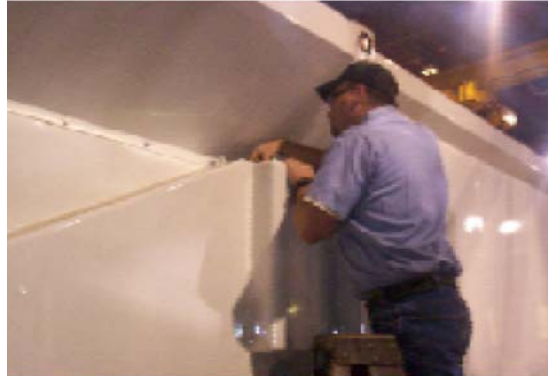
Figure 3-28 Proper position to adjust pendulum proximity switches
