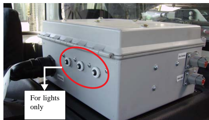
Figure 3-13 Auto-reset circuit breakers
