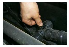
Figure 184. Sampler coupler
