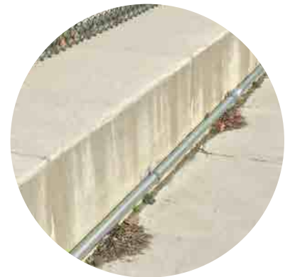
ELECTRICAL CONDUIT ALONG FOUR MILE RUN TRAIL
