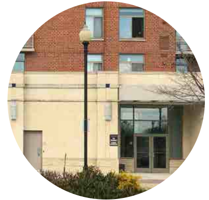
EXISTING POLE LIGHTS
