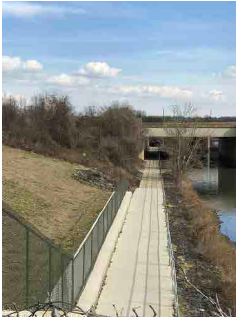
2. View of Four Mile Run Trail from Route 1 toward Potomac Avenue.
