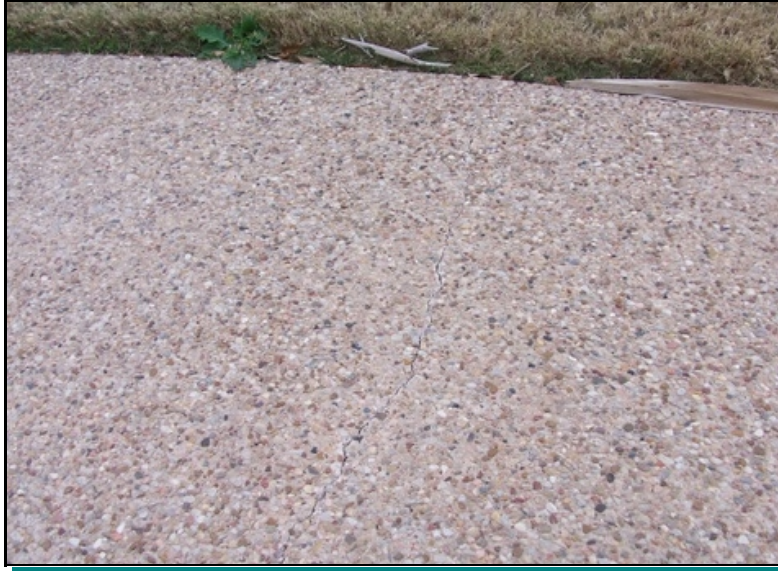
Crack in concrete sidewalk
