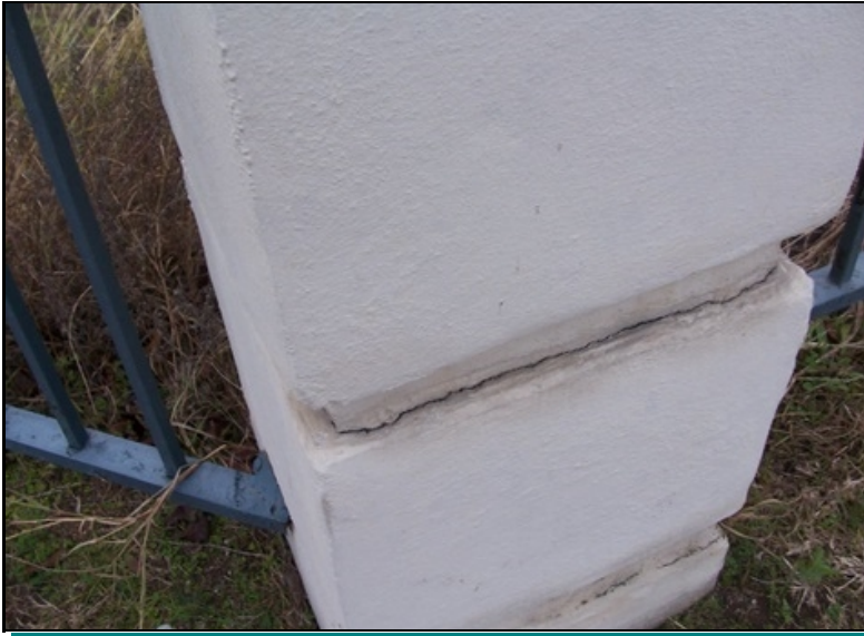
Crack at stucco finish
