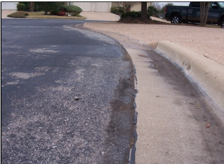
Isolated pavement settlement near gutter
