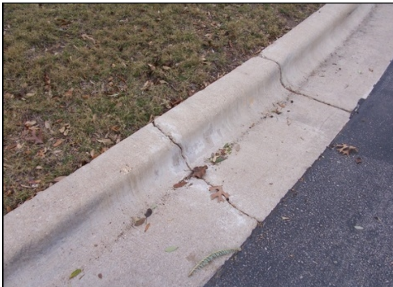
Crack in concrete curb
