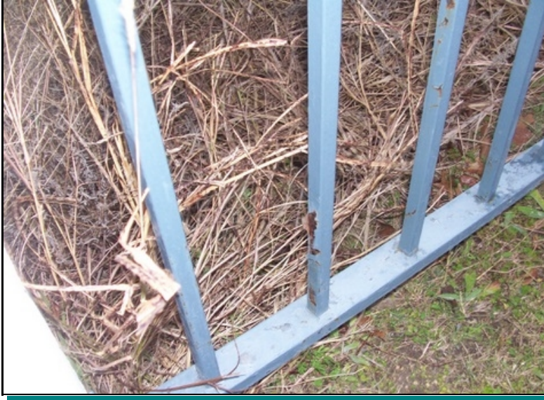
Rust and paint finish deterioration
