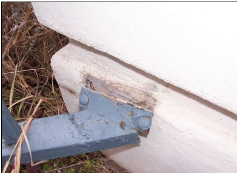
Loose connection at fence and column
