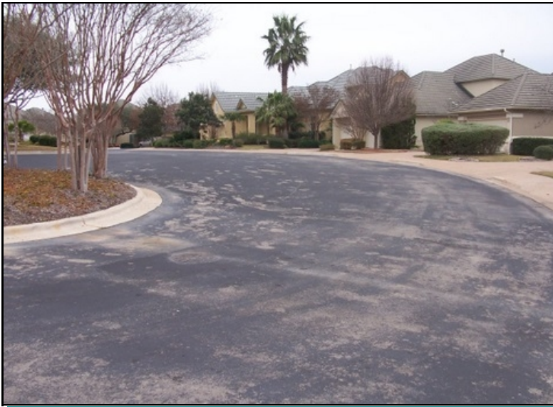
Worn seal coat at pavement
