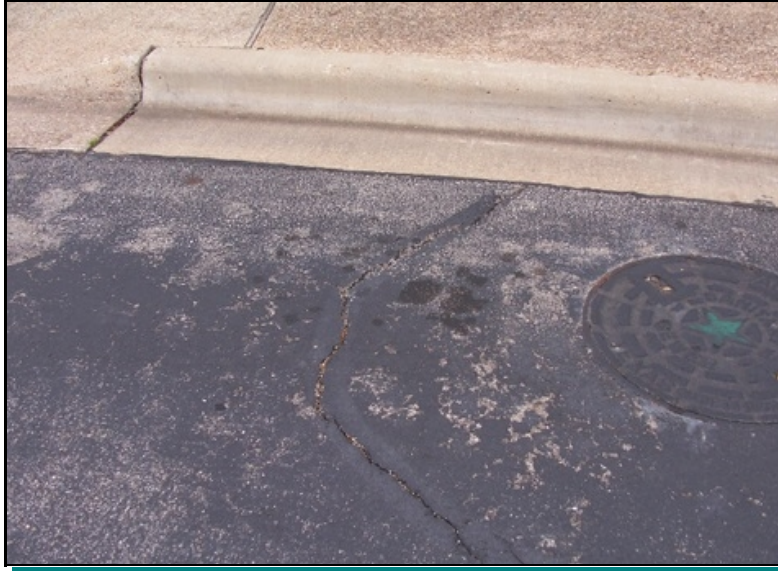
Isolated crack in pavement
