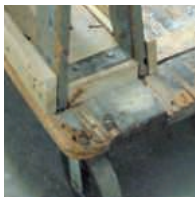
Wood—splinters and rots
