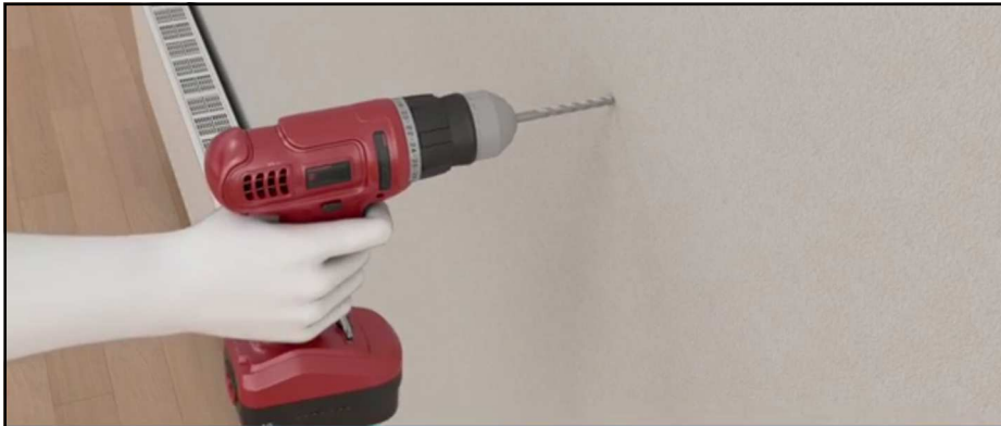
Drilling through cables
