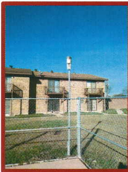
Swimming Pool North Side Light / Poles
