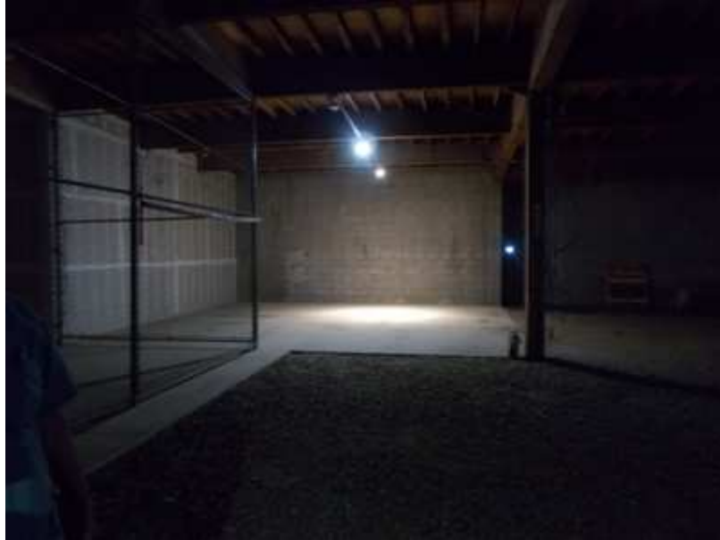
The Warehouse Area is unfinished. Complete Rehab of the Warehouse has not been included in the Study.
