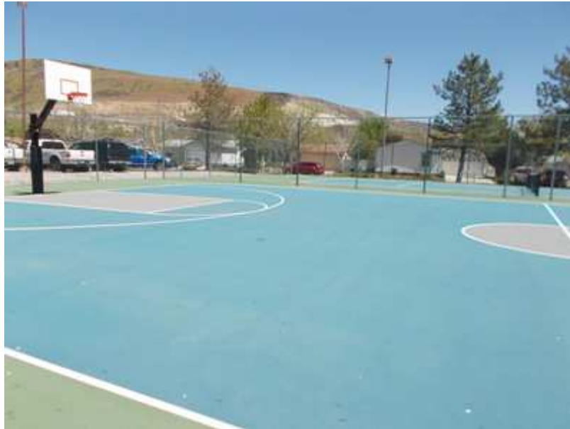
The Tennis Court Resurface, Sealing, Basketball Hoops and Chain Link Fencing have been included in the Common Area Category.
