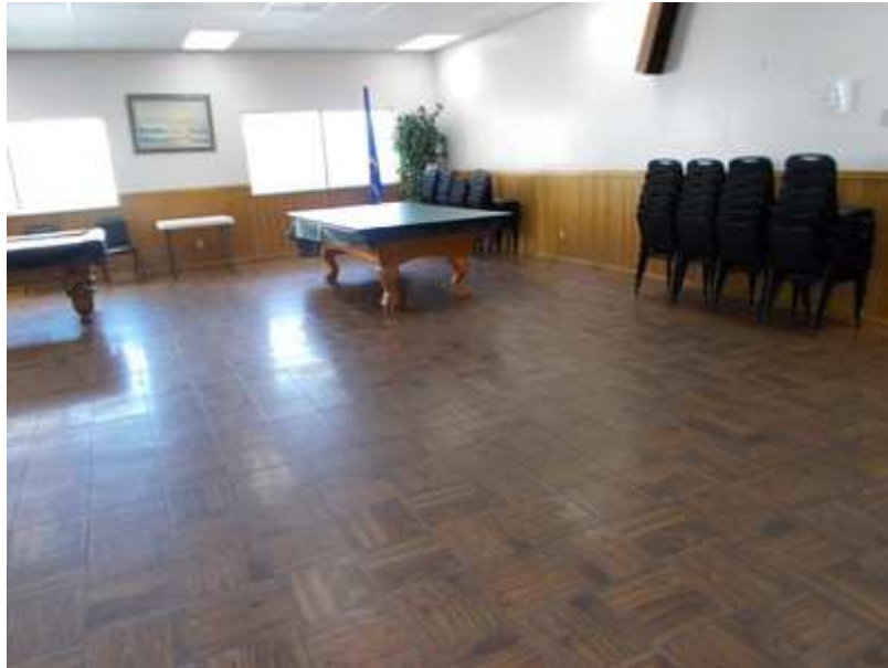
The Community Room Flooring, Pool Tables, Furniture, Painting and Lighting and Electrical have been included as components in the Study.
