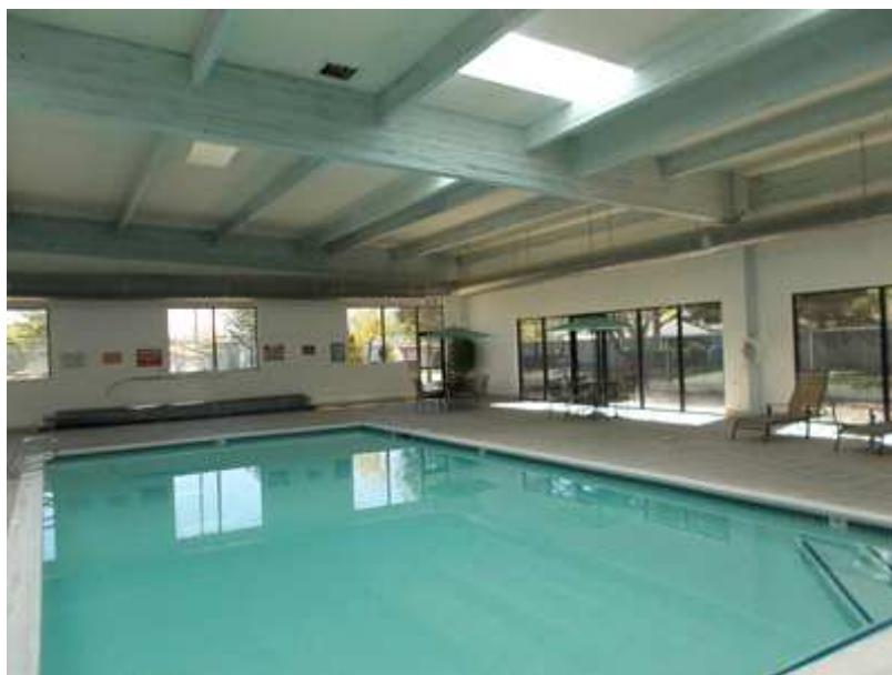
The Pool Area Components include Pool Concrete Deck, Pool Furniture, Pool and Spa Re-Surface, Heater, Pump, Pool Cover Interior Painting, Filter Replacement and Ventilation System. The Useful Life of each component is an estimation only.
