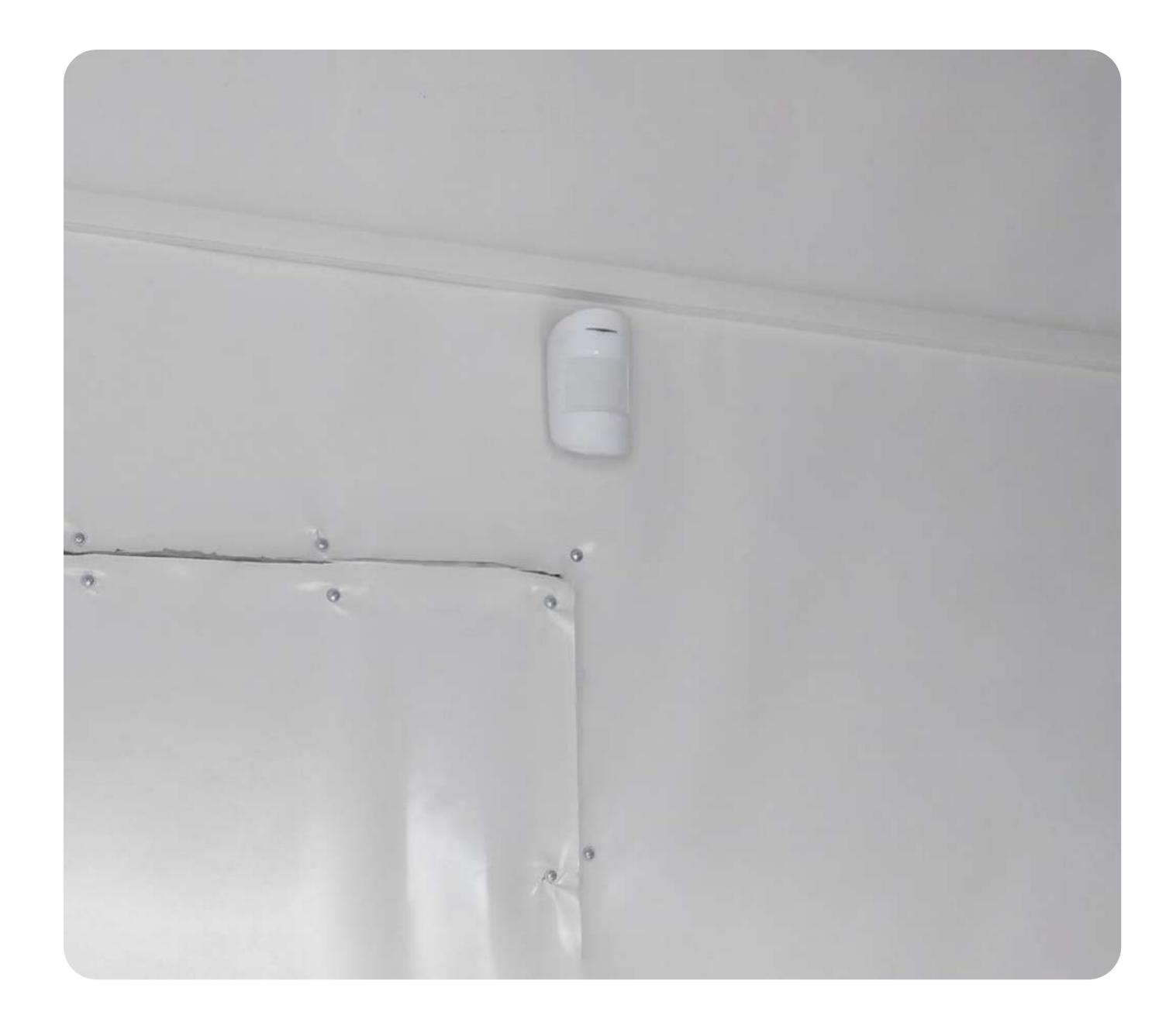
Thus, the MotionProtect motion detector backs up the DoorProtect opening detector. It is common practice for one detector to verify the triggering of another detector to eliminate false alarms. On the farm, notifications are turned on when each of the detectors is triggered. Even if an intruder enters the greenhouse not through the door, they will not hide from the motion detector.
