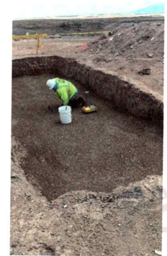
Compaction testing per georeport
