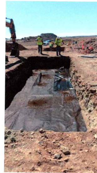
Geo fabric placement per georeport
