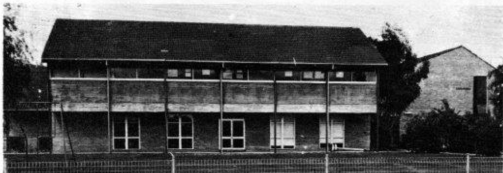
The school as it is today. This is the front view of a modern complex.
