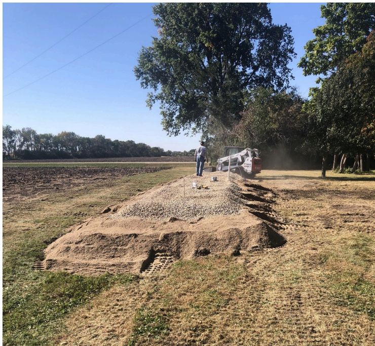
Figure 2. Septic system replacement mid-completion.
