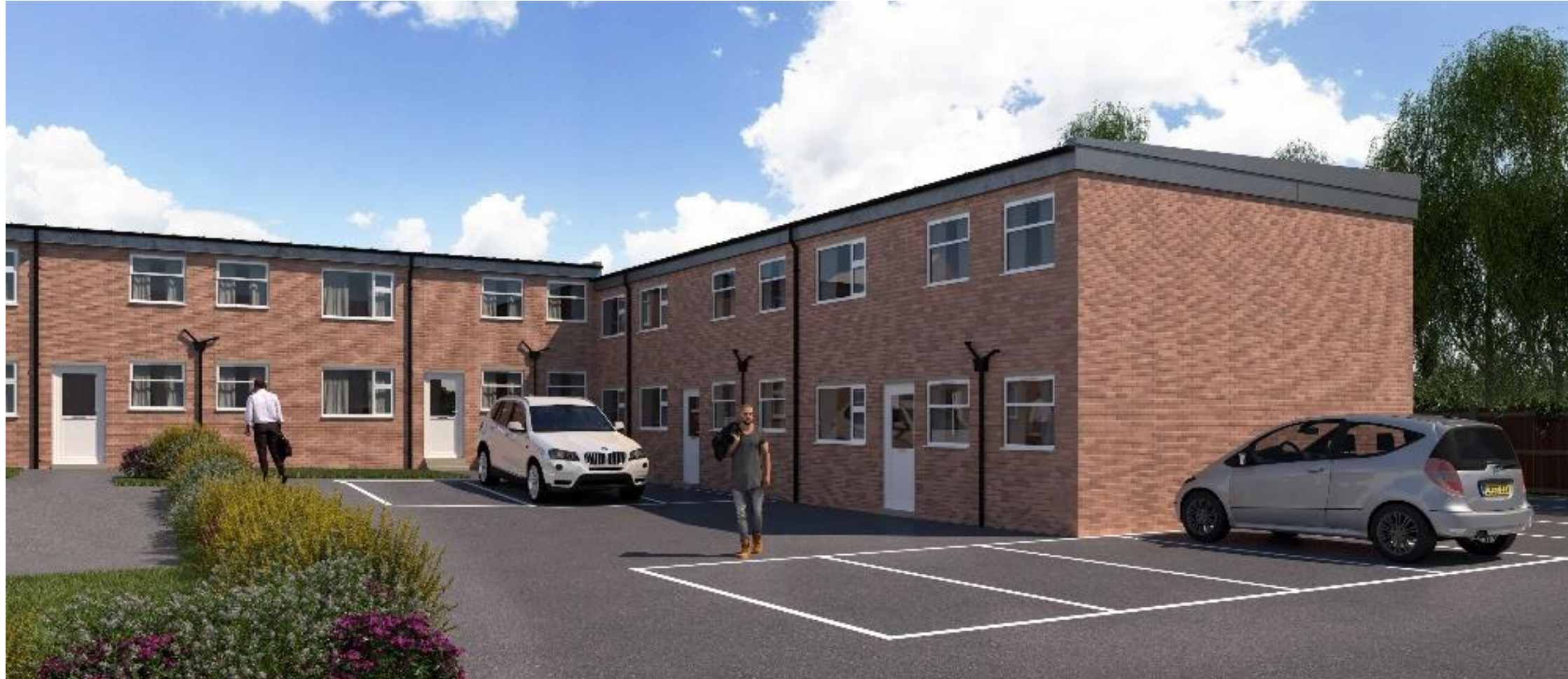
St. George's Courtyard (St George's Courtyard Ltd)
