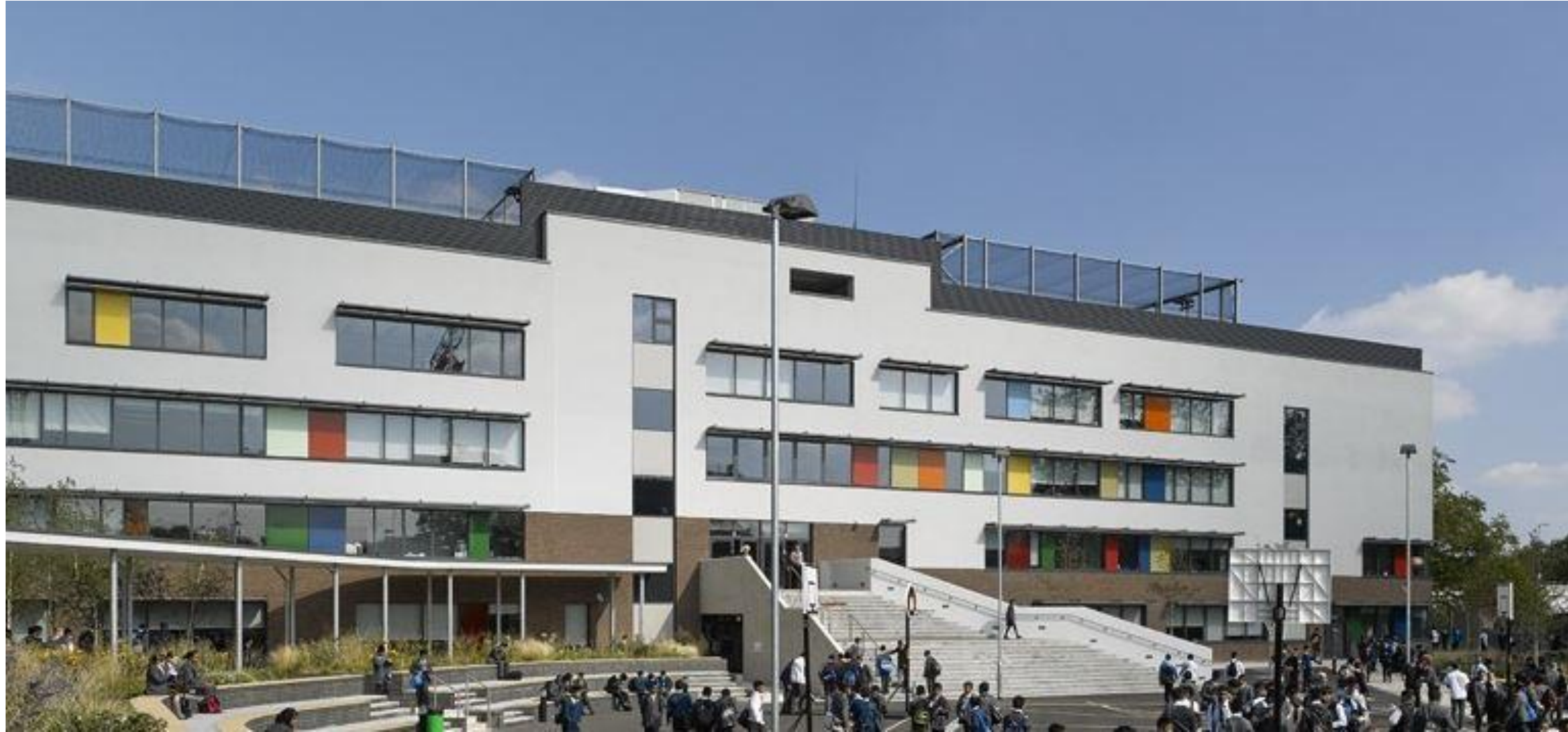
Bow School (Bouygues UK)
