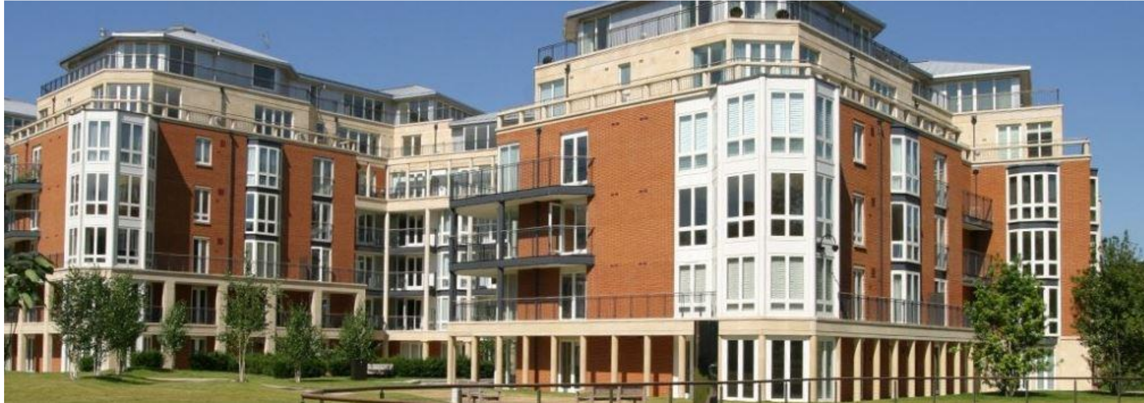
552 Kings Road (Bouygues UK)
