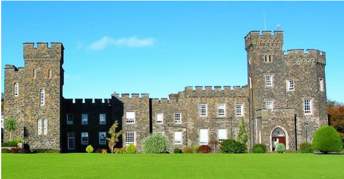
Garron Tower, Carnlough, County Antrim today.
