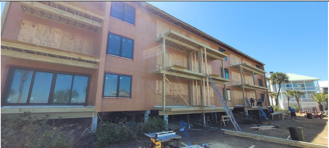
DECK FRAMING / DOOR AND WINDOW INSTALL PROGRESS 3-25-2025
