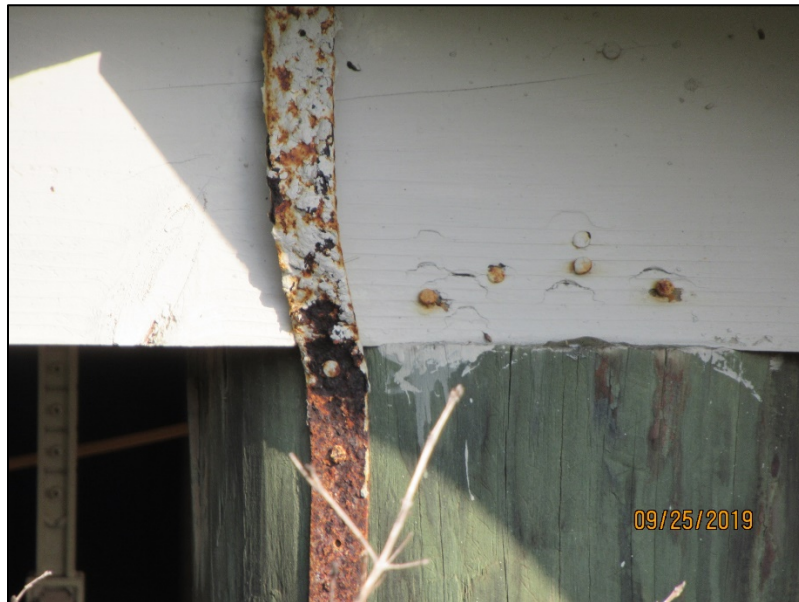
Typical corroded metal strapping at piling.
