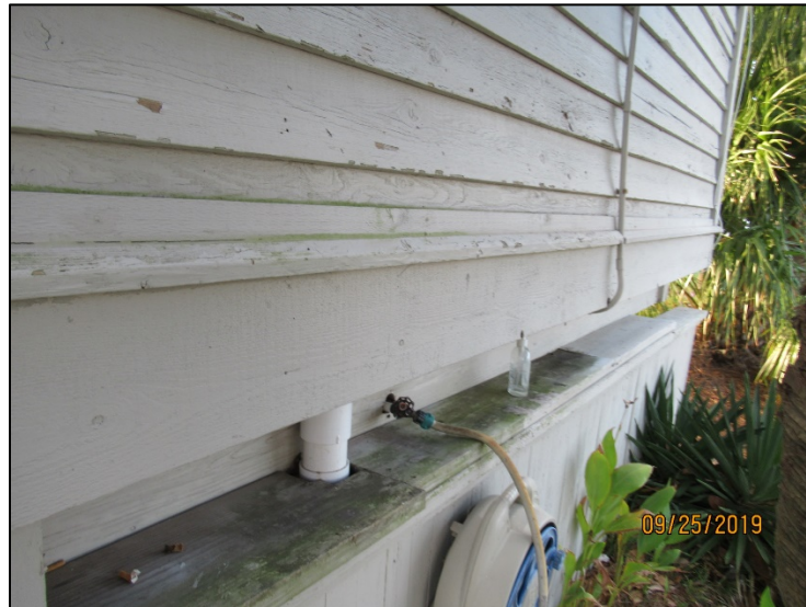
Typical condition of wood siding with peeling, pitting and deterioration of horizontal wood fibers.
