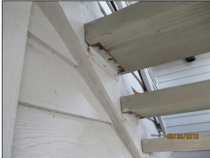
Corroded steel tread bracket
