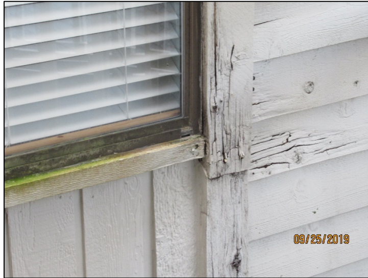
Typical deteriorated window trim and siding near “light well”
