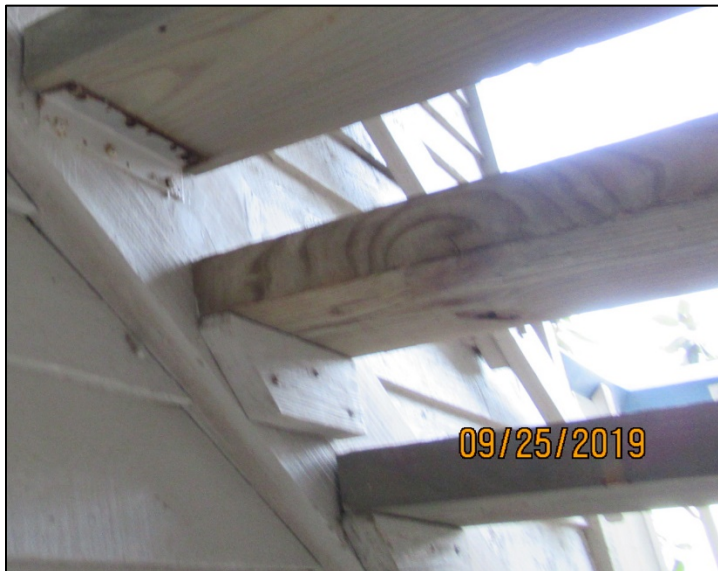
Mitered 2x4 tread bracket and typical steel tread bracket
