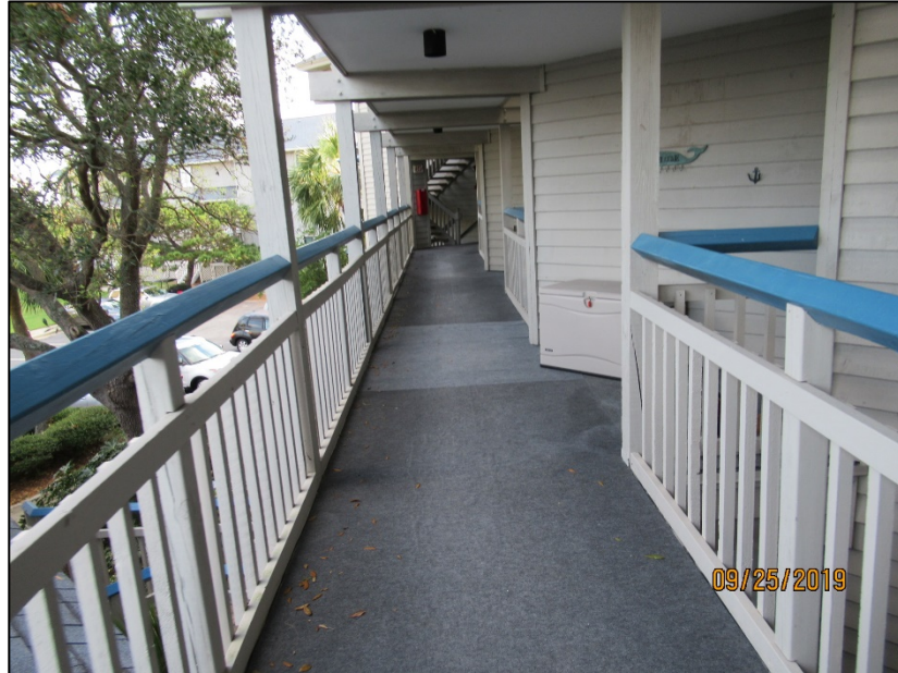
Typical walkway, note various replacements and water staining currently on carpet surface
