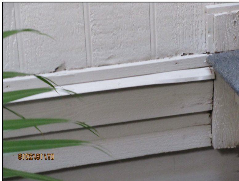
Siding and trim deterioration
