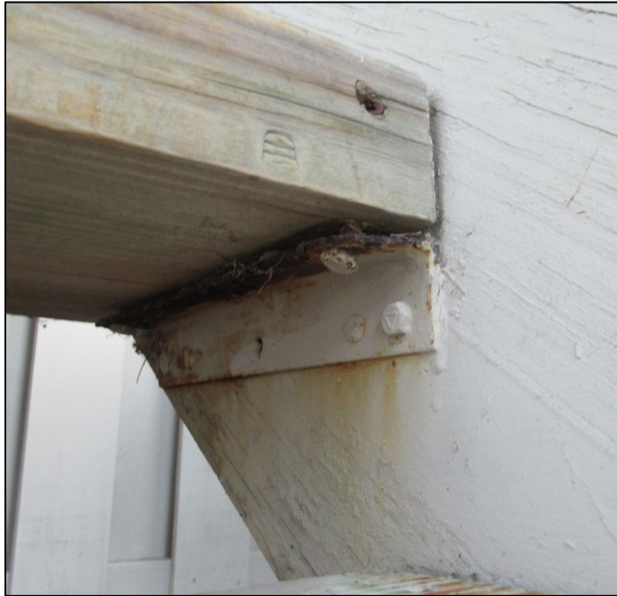
Corroded steel tread bracket
