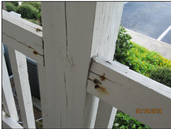
Upper rail of guardrail deterioration
