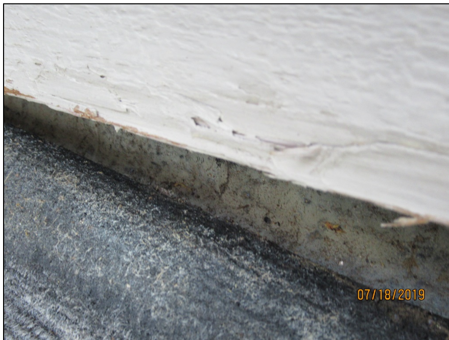
Wall/walkway transition with no continuous flashing up the wall
