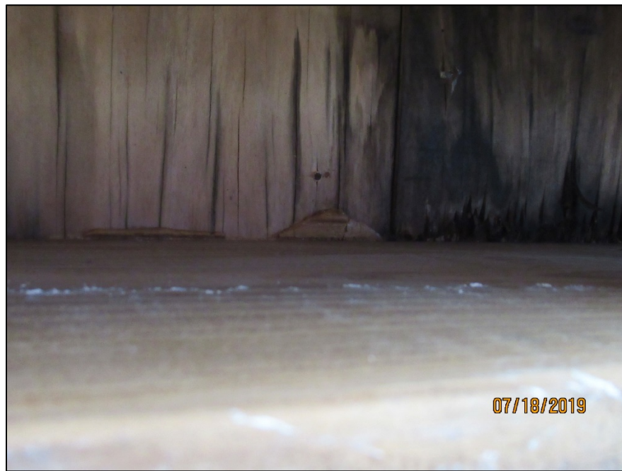
Underside of deteriorating decking as viewed from level below
