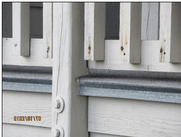
Guardrail deterioration
