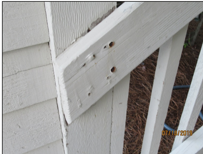
Handrail connection, deterioration
