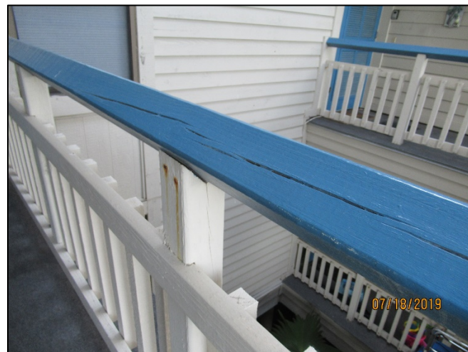
Top rail of guardrail deterioration
