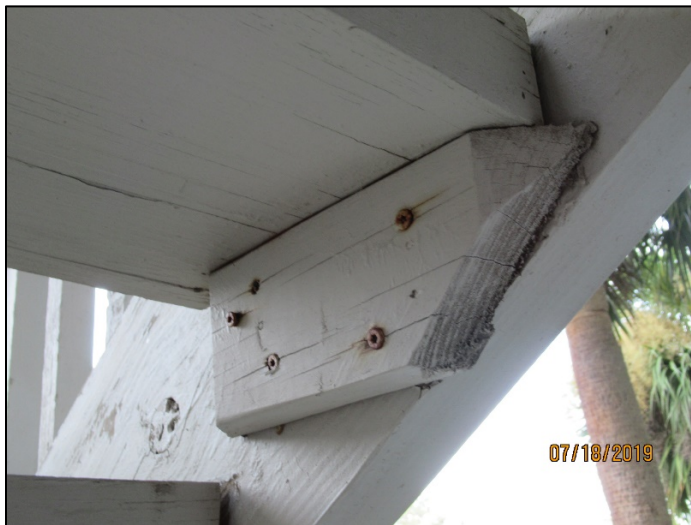
Mitered 2x4 tread bracket
