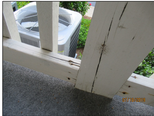
Lower rail of guardrail deterioration
