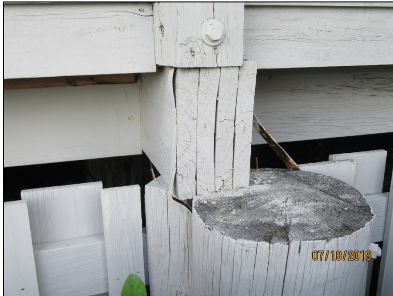
Misaligned framing at piling and corroded strapping.
