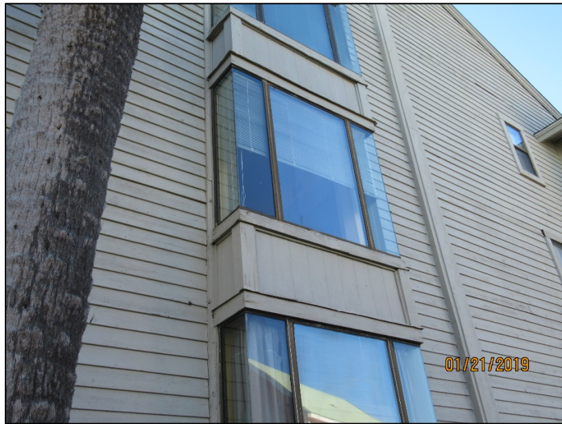
Typical “box bay” window with corner glass
