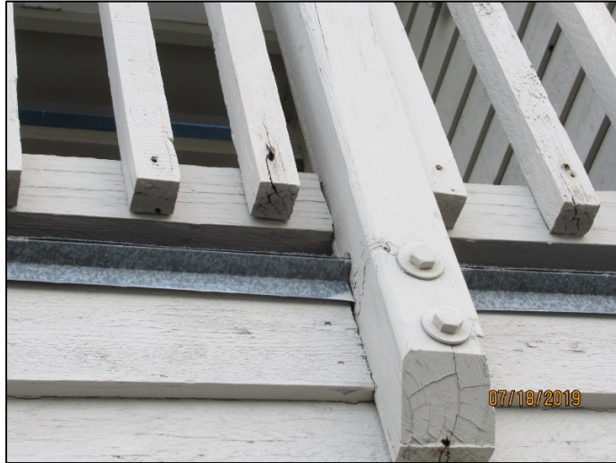
Guardrail deterioration
