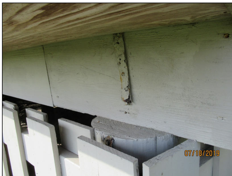
Corroded/missing strapping at piling
