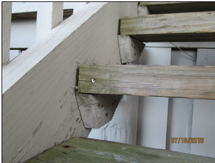
Mitered 2x4 tread bracket
