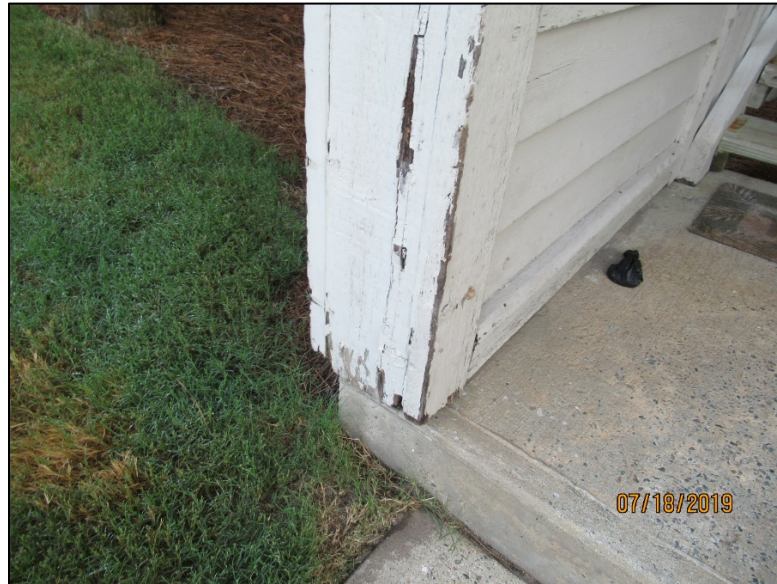
Wood trim deterioration
