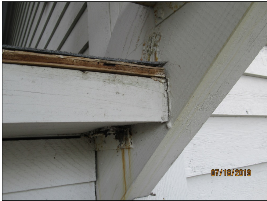
Deteriorated and delaminating walkway decking
