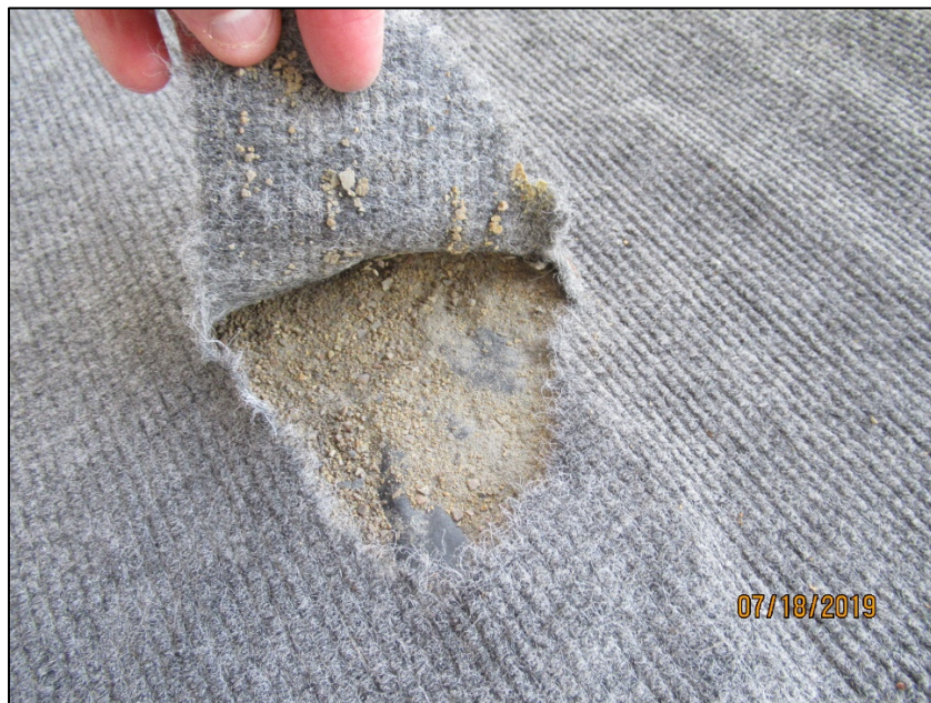
Tear in Third floor walkway carpeting exposing rippled water-resistant membrane
