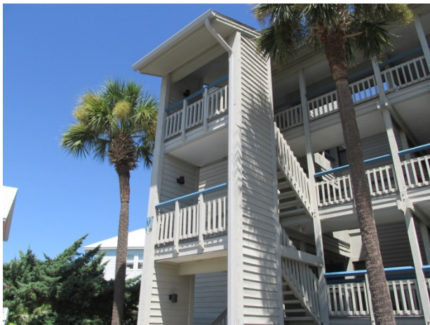
Staircases at Building M
