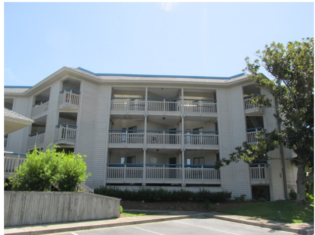
Building L overview
