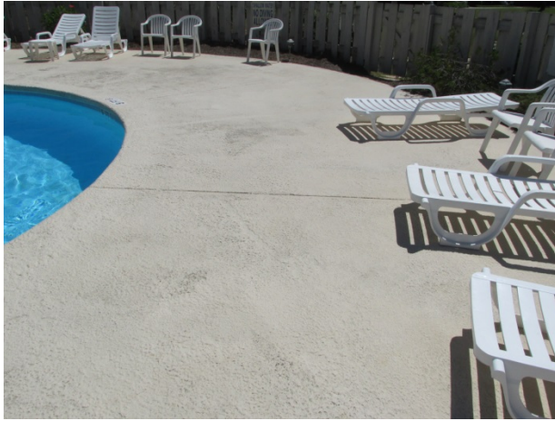
Concrete deck overview
