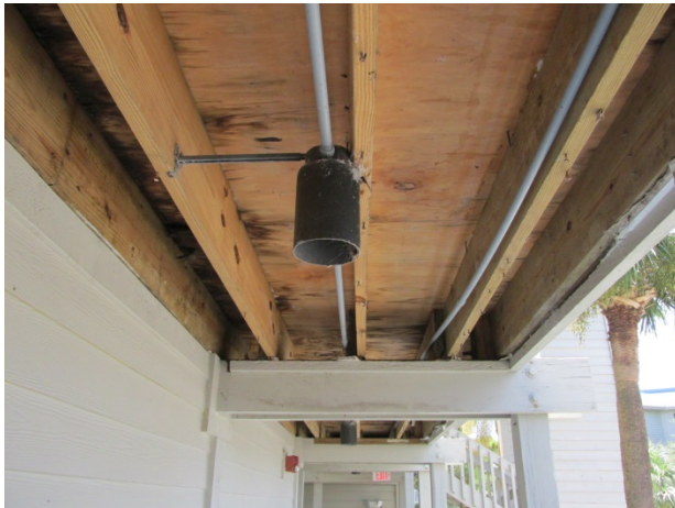
Wood soffit being replaced
