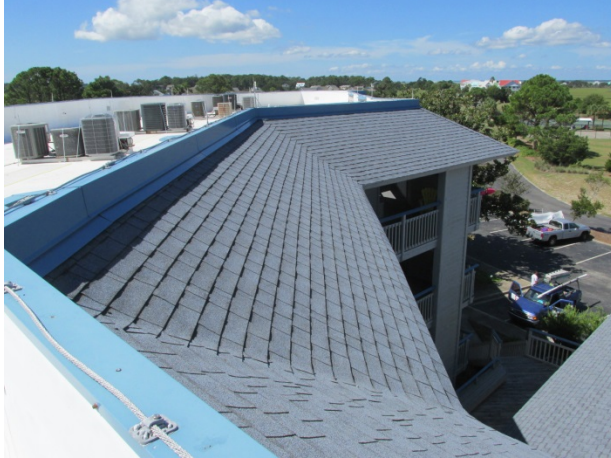
Asphalt shingle roof overview
