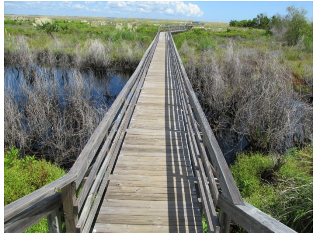
Boardwalk in good condition
