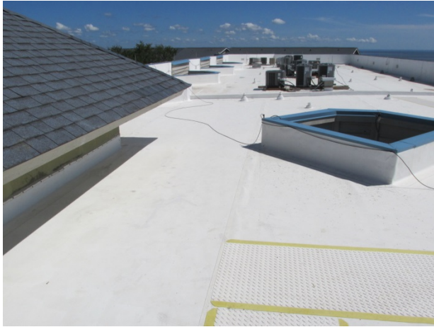
Thermoplastic roof overview
