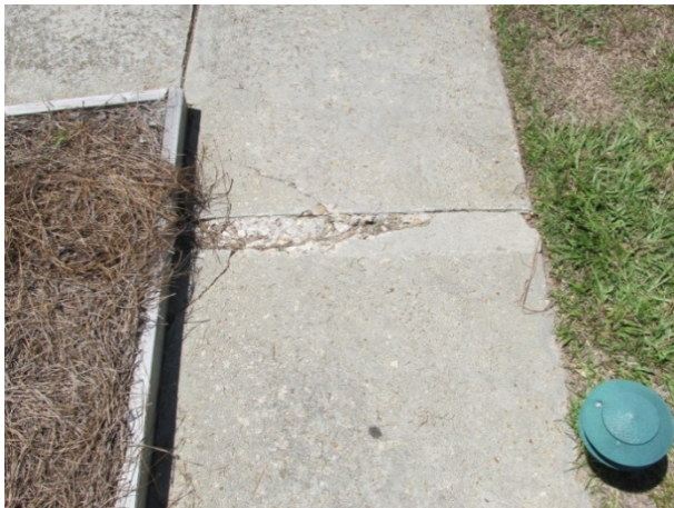
Isolated cracks
