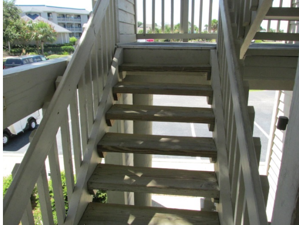
Stairs in good condition
