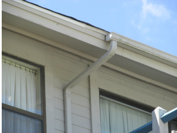
Typical gutter and downspout assembly
