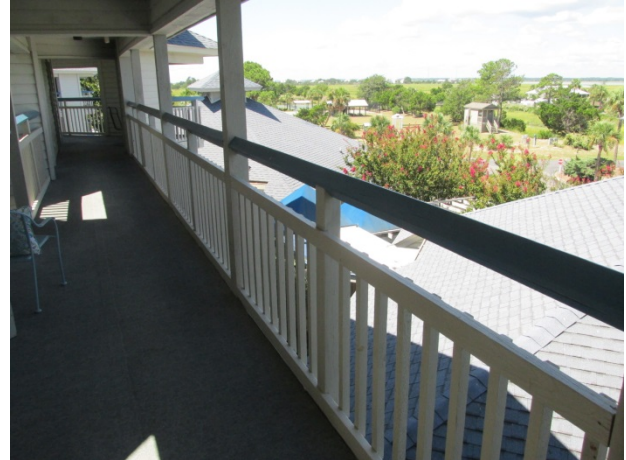
Wood railings in good condition
