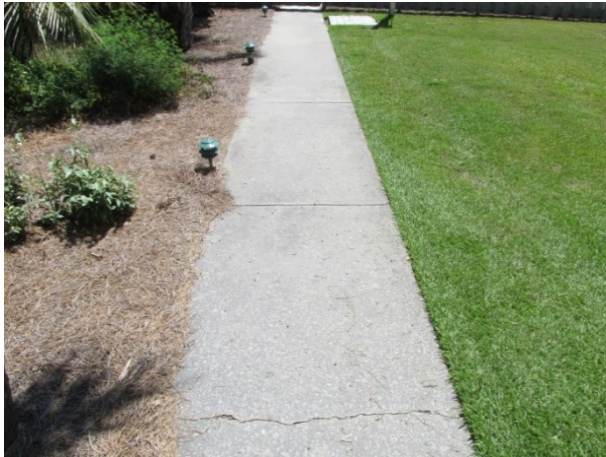
Concrete sidewalk overview
