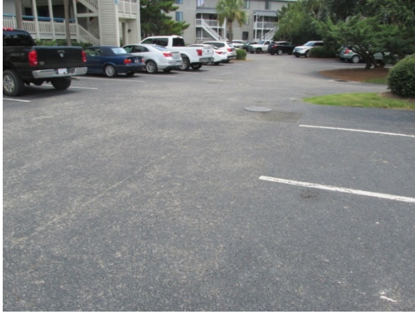
Asphalt pavement overview
