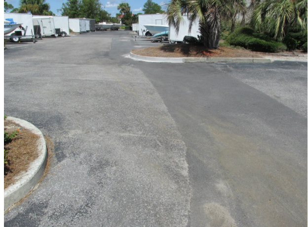
Replaced section of asphalt pavement
