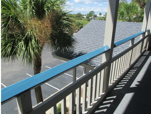
Wood railing overview
