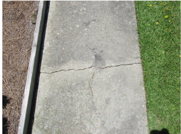
Isolated cracks
