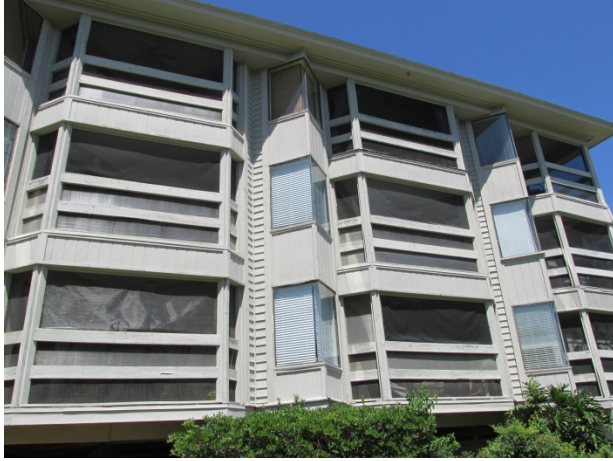
Screens at the balconies
