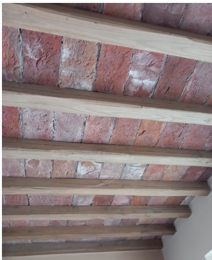
The ceiling made with salvaged tiles
