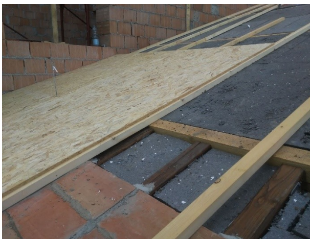
Waterproof bitumen membrane above the air chamber
