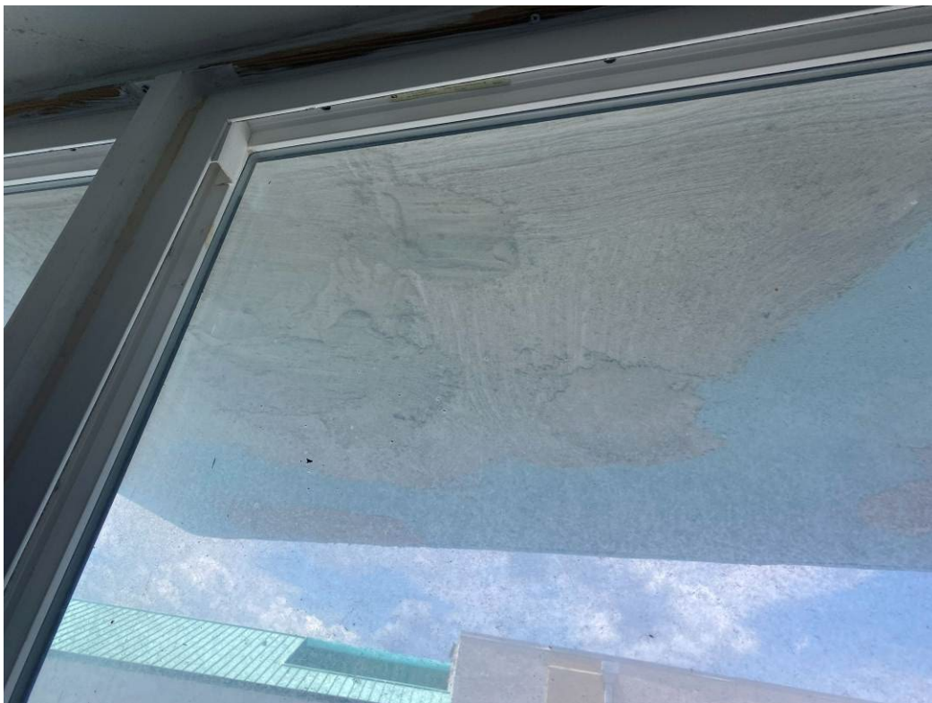
Photograph #18 – Typical ceiling concrete spalling
