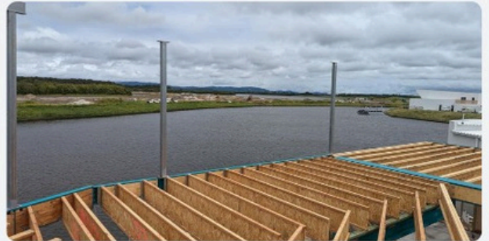
Deck & Structure Framing
