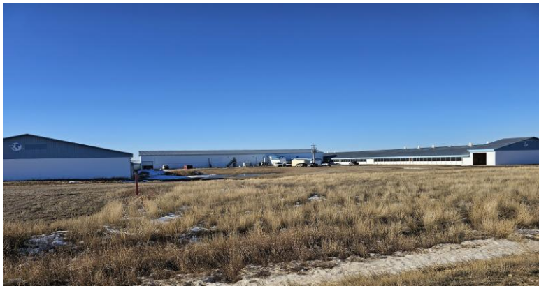
Agricultural Production facility: 2.5MW PPA 19 acre site, 5MW capacity grid connection Operating wind farms are located to the west, south, and north
