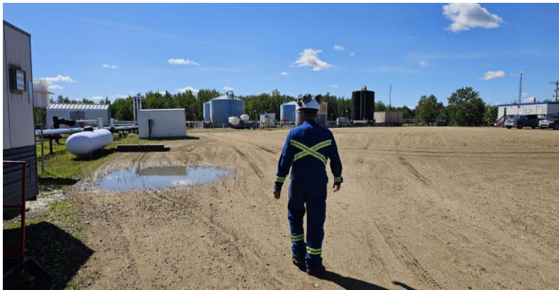
Oil battery: 2.5MW PPA 4 acre site, 5MW capacity grid connection
