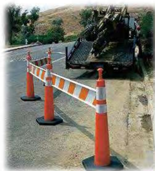
Channelize traffic with 42" Grabber-Cone and optional plastic barricade panels
