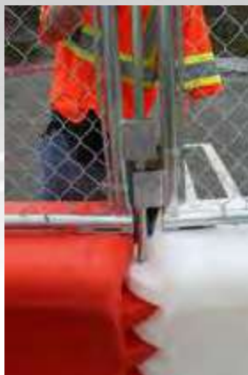
T-Pin Connects Wall to Fence
