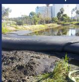
Implemented a cofferdam to create a dry dock and install a self-gravity pump station and transfer to filtered vaults.
