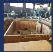
Constructed a robust foundation using 100 cubic yards of concrete to provide structural support for a 250,000 lbs press.
