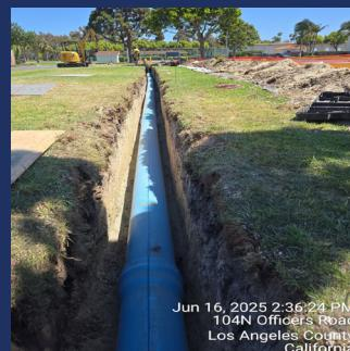
Installed approximately 400 linear feet of 12-inch PVC water main to service buildings. Scope included trenching, backfill, disinfection, eight new service laterals, safety controls, system cutover, and full surface restoration.
