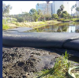
Implemented a cofferdam to create a dry dock and install a self-gravity pump station and transfer to filtered vaults.
