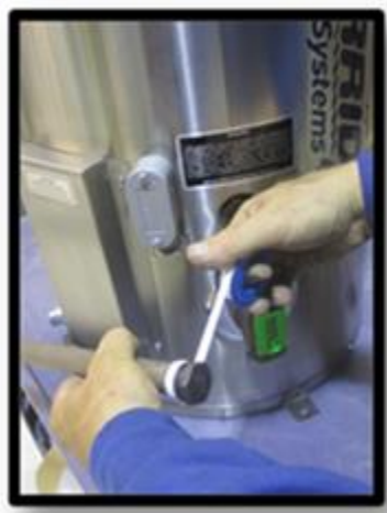
Image 1.3 Install new anode with PTEF tape or similar sealant.
