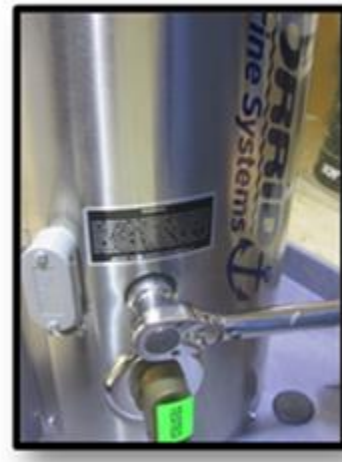
Image 1.2 Remove anode with 1-1/16" socket.
