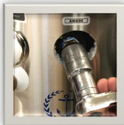
Image 1.2 Remove anode with 1-1/16" socket.
