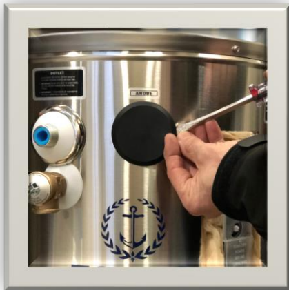
Image 1.1 Locate anode and remove plastic cover.
