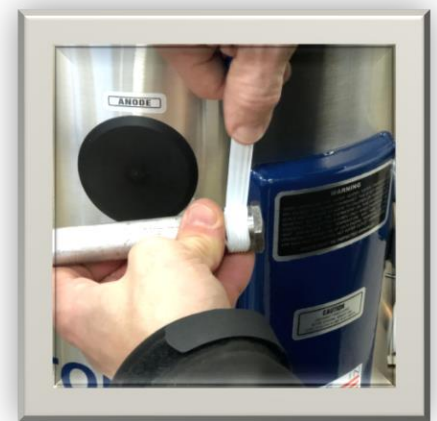
Image 1.3 Install new anode with PTEF tape or sealant.
