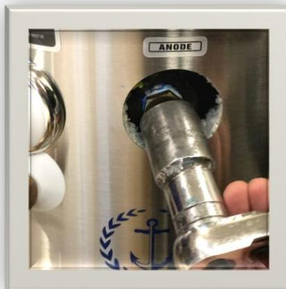
**Image 1.2** Remove anode with 1-1/16" socket.
