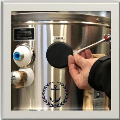
**Image 1.1** Locate anode and remove plastic cover.
