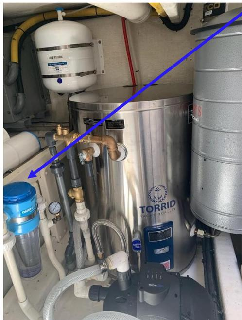
A Calcite Buffer is recommended when using reverse osmosis water makers. The RO water is slightly acidic. When it enters the water heater, it tries to balance back to PH neutral by re-mineralizing from the anode. If anode is depleted, it will attack the fittings next.
